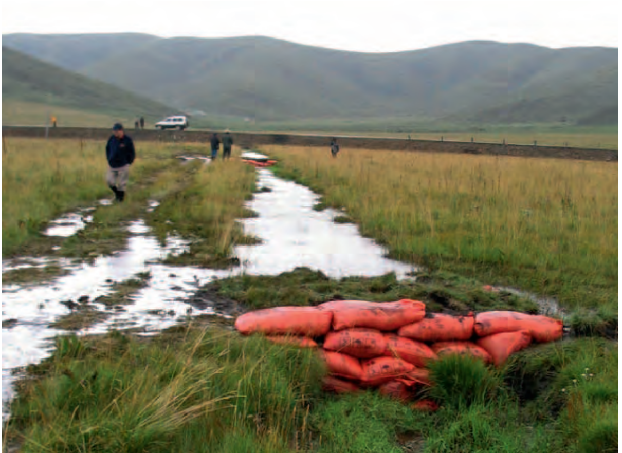
Blocking erosion gullies helps to restore the water storage capacity of the Ruoergai (China) peatlands. By Chen Kelin
